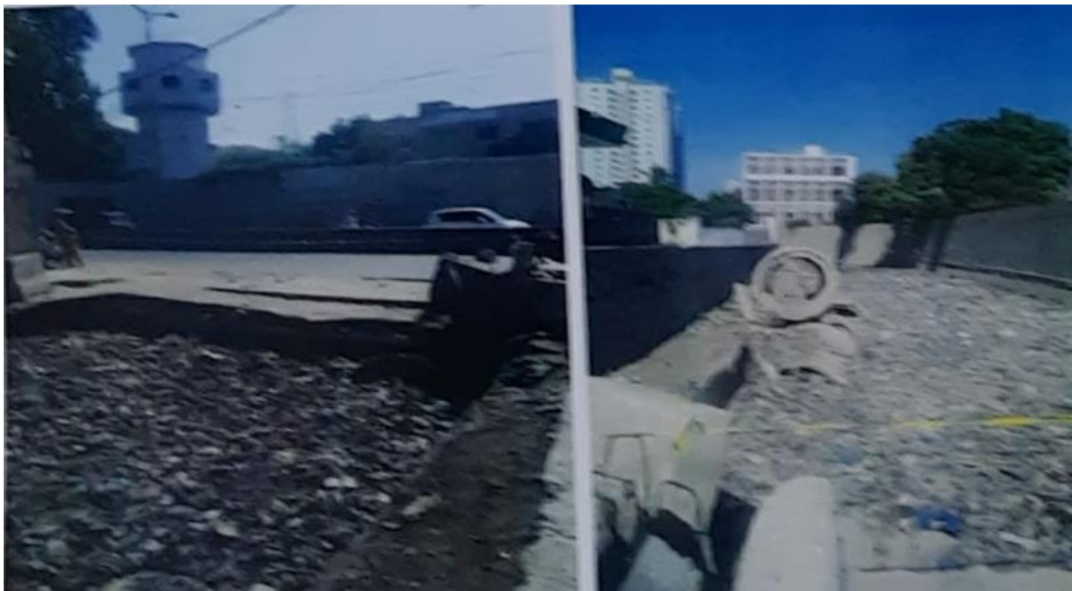
iii. Drain near police headquarter
